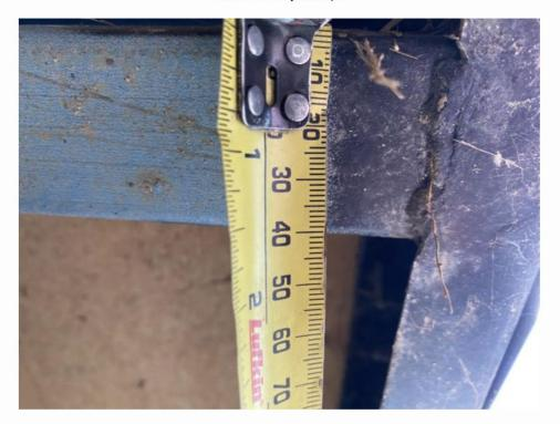
Photo 2: Floor joist width
