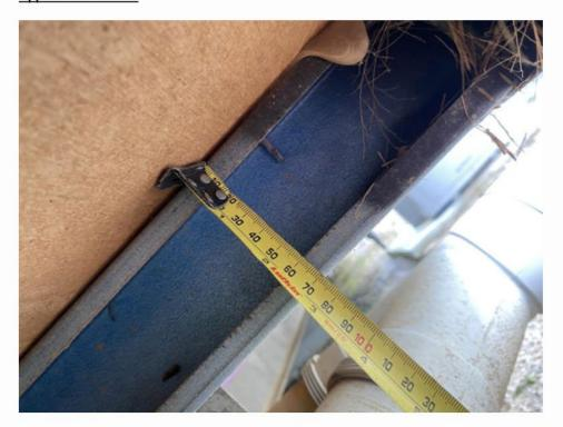
Photo 1: Floor joist depth
